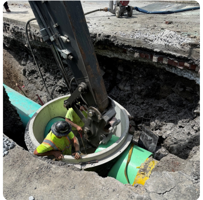
Cross Street Phase II Completion, City of Troy
