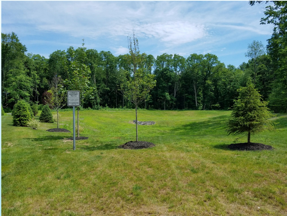
Stormwater Infiltration Basin
