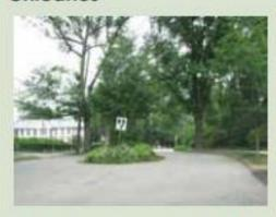
A series of narrowings or curb extensions that alternate from one side of the street to the other forming S-shaped curves can be implemented to reduce motor vehicle speeds and unlock roadway space
