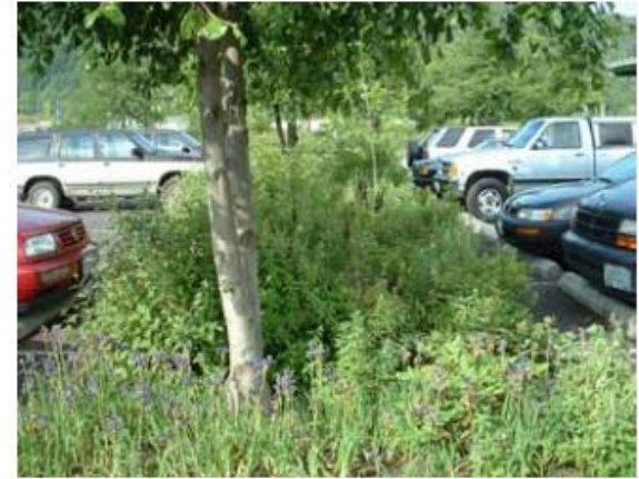
Figure 6. This landscape area is designed to accept and treat stormwater runoff in this Portland, OR parking lot
