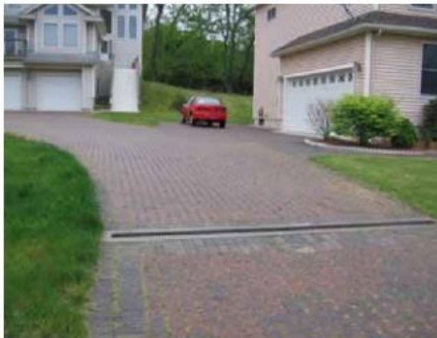
Figure 11. This shared driveway in Jordan Cove, CT helps to reduce impervious cover and is also constructed using permeable materials.
