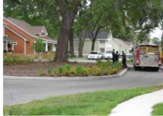
Figure 4. Road widths are minimized in this Savannah, GA neighborhood; yet are wide enough to allow access for emergency vehicles
